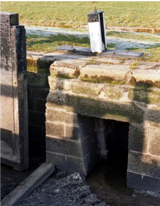
Four types of ground paddle used on the canal. Top left is an up-and-over type, here on the Bank Newton locks. Top right is an open frame box paddle found on the Rufford branch. Bottom left is a sloping box paddle as found at Barrowford and Gargrave, with bottom right a vertical box paddle with brake lever used at Greenberfield.
