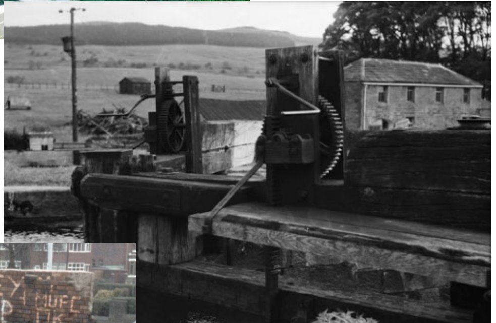
Lancashire jack cloughs, such as here at Poolstock, were slightly different, although both had to be worked from a platform fitted to the side of the gate. These are now considered dangerous, and none survive. The paddle opening size was increased in the 1850s to speed passage through the locks, and counter balances were provided to make them easier to operate.
