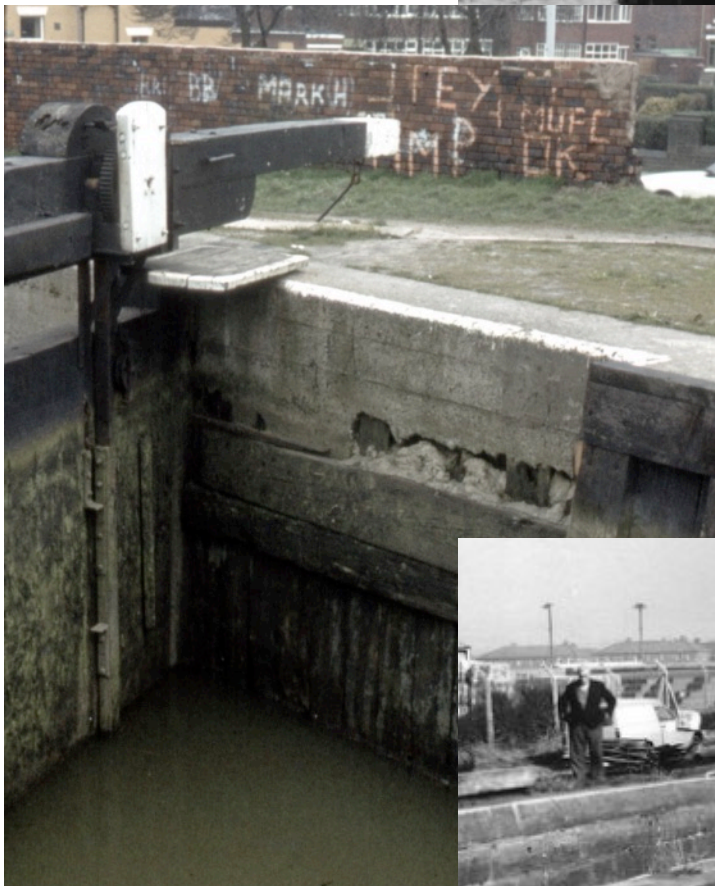
Lancashire jack cloughs, such as here at Poolstock, were slightly different, although both had to be worked from a platform fitted to the side of the gate. These are now considered dangerous, and none survive. The paddle opening size was increased in the 1850s to speed passage through the locks, and counter balances were provided to make them easier to operate.
