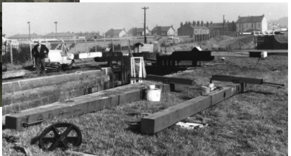
Lancashire jack cloughs, such as here at Poolstock, were slightly different, although both had to be worked from a platform fitted to the side of the gate. These are now considered dangerous, and none survive. The paddle opening size was increased in the 1850s to speed passage through the locks, and counter balances were provided to make them easier to operate.
